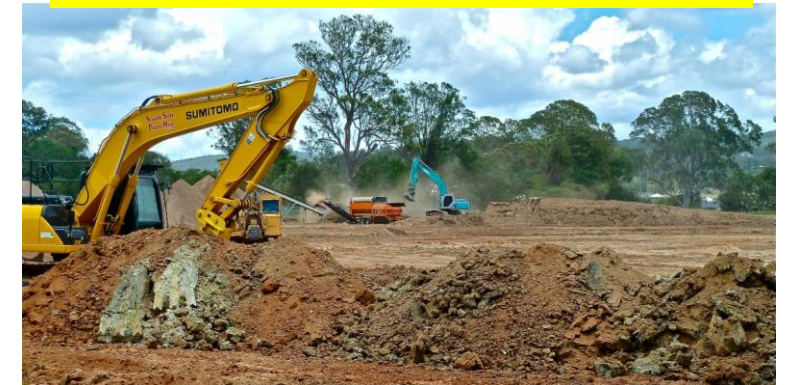
Construction on Farm Land
