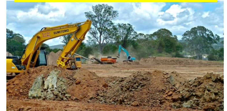
Construction on Farm Land
